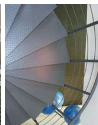
Bottom right: Chequer plate steel treads on a large commercial spiral stair.
